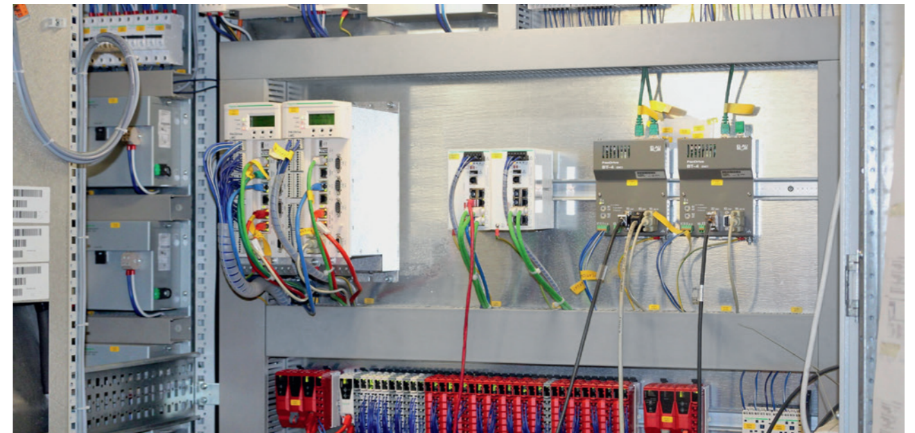
Figure 3: The entire system is controlled with two PacDrive 3 LMC controllers operating in parallel, below are two safety controllers with a mixed I/O field.
