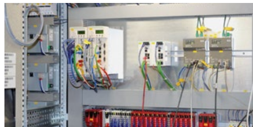
Figure 3: The entire system is controlled with two PacDrive 3 LMC controllers operating in parallel, below are two safety controllers with a mixed I/O field.
