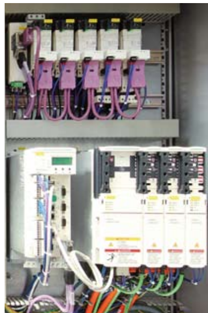
The PacDrive 3 automation solution: The new LMC-series controller is on the left, next to it on the right is the shared power supply with LXM 62 servo drives arranged upon it; above this, a row of TeSys U motor starters
